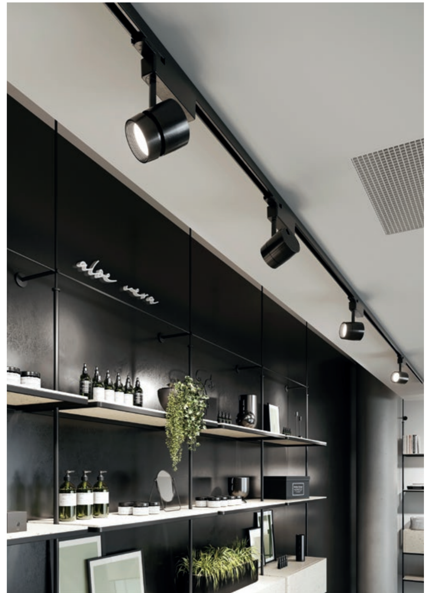
The use of the Expo Adjust system in a beauty supply boutique.
